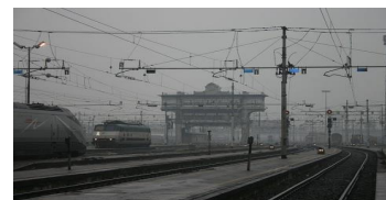
Railway - voice / data communications services
